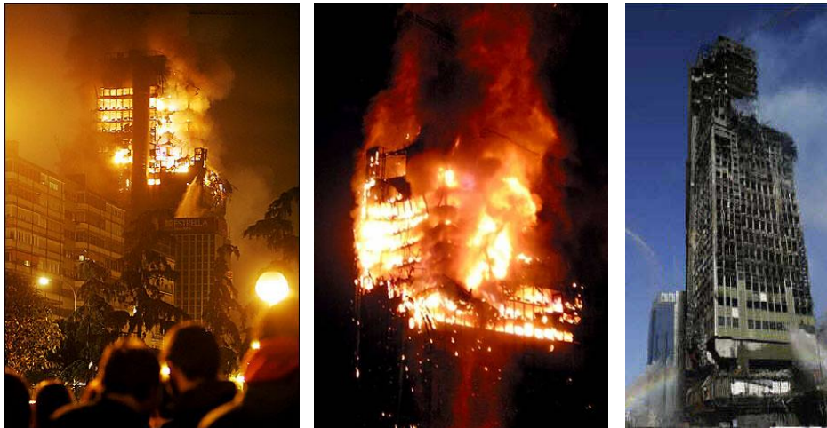
Figure 2-10 Windsor Building on Fire and post Fire
