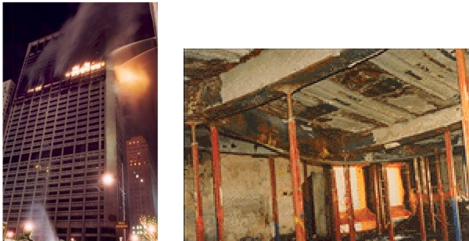
Figure 2-3 One Meridian Plaza on Fire and post Fire
