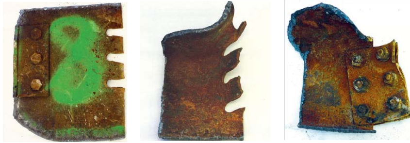
Figure 2-8 Failed Bolt Connections from WTC 5 (FEMA 403)
