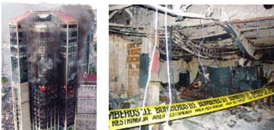
Figure 2-9 Caracas Plaza Fire and Fire Damage on Floor
