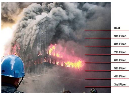
Figure 2-4 WTC 5 on Fire (FEMA 403);
